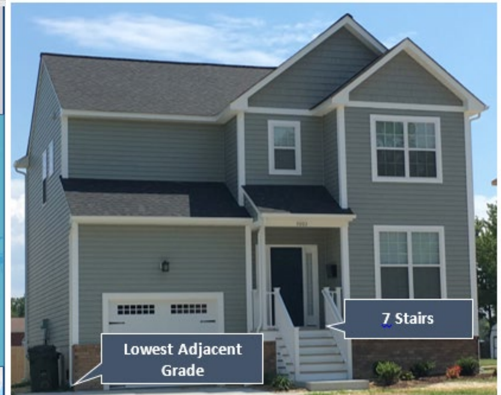
Figure 3: Illustration of stair counting approach for estimating FFH. The count of 7 stairs equals a FFH of 4.4ft. The land elevation difference between the bottom of the stairs and lowest adjacent grade would be added to produce the final FFH estimate. Image from City of Hampton Property Information Parcel Viewer (2017).
