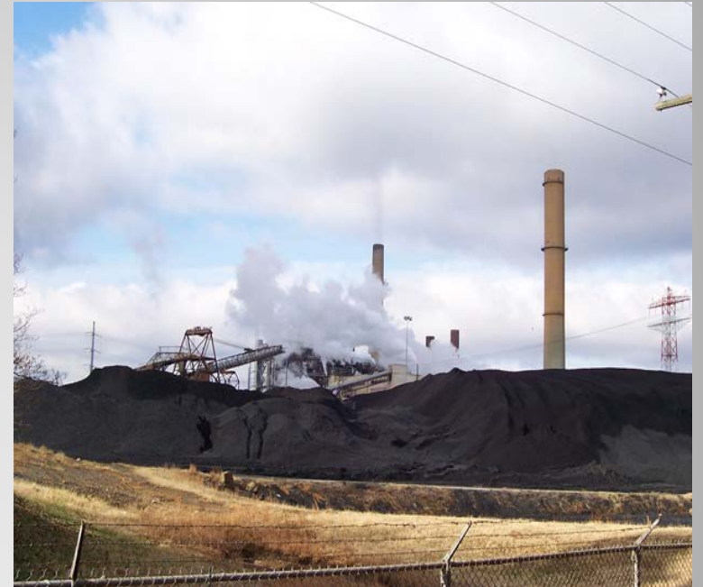
Dominion Power Station in Chesterfield, VA
