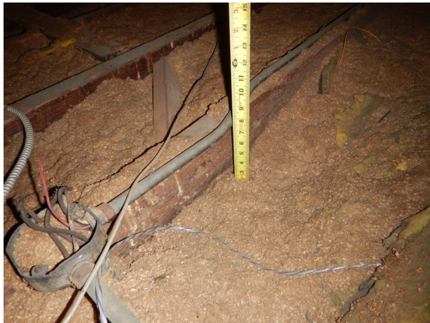
Before Picture of Attic
