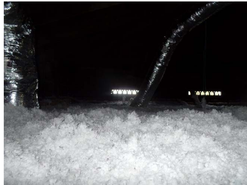
Post Retrofits Picture of Attic
