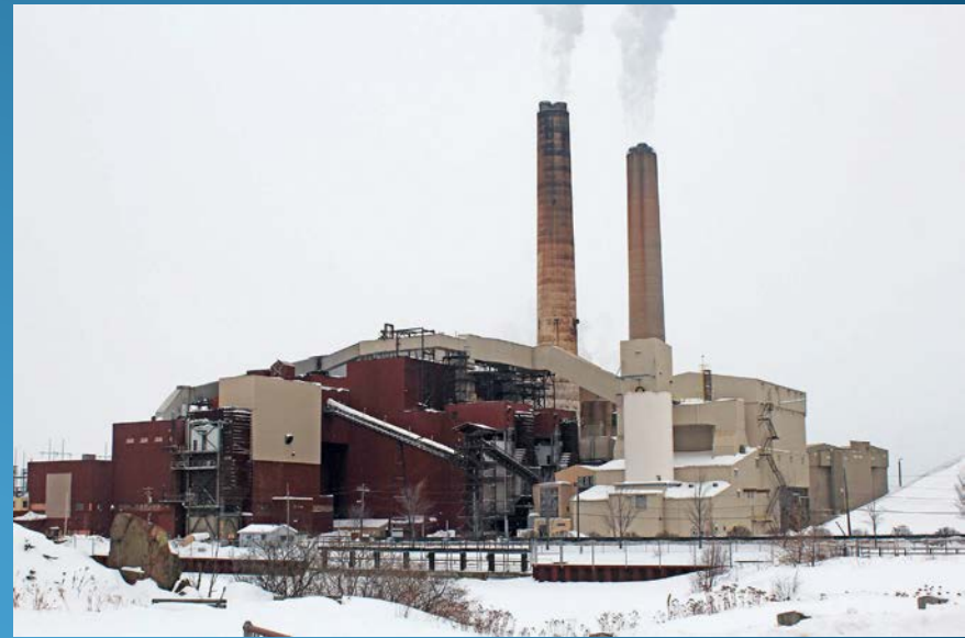
Old Coal Plant
